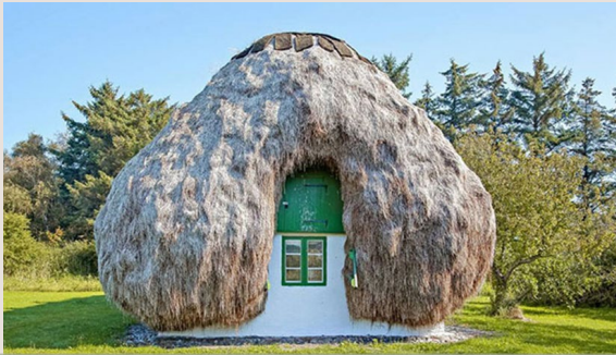
Figure 25. Zostera marina leaves used as roof thatching for a historic farm on the island of Læsø.
